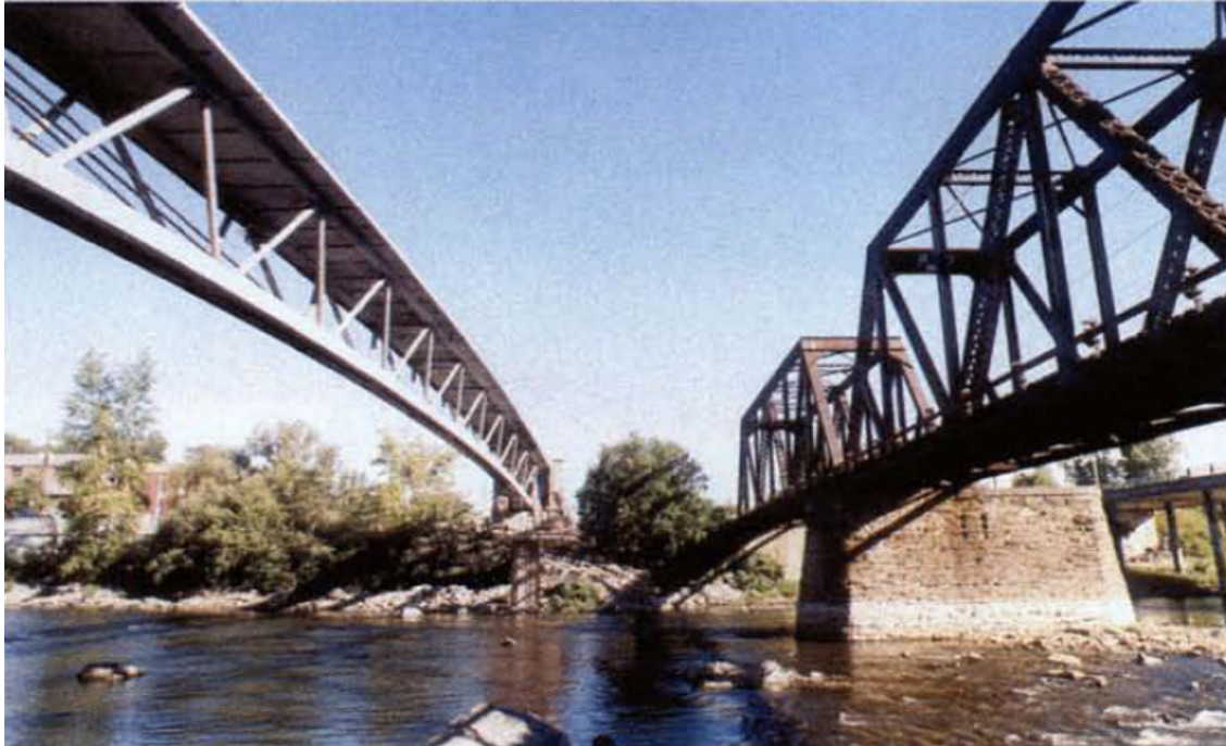
Figure 2.6: Comparison of the new UHPC Sherbrooke Footbridge (left) and a Steel Truss Crossing (Blais & Couture, 1999)
