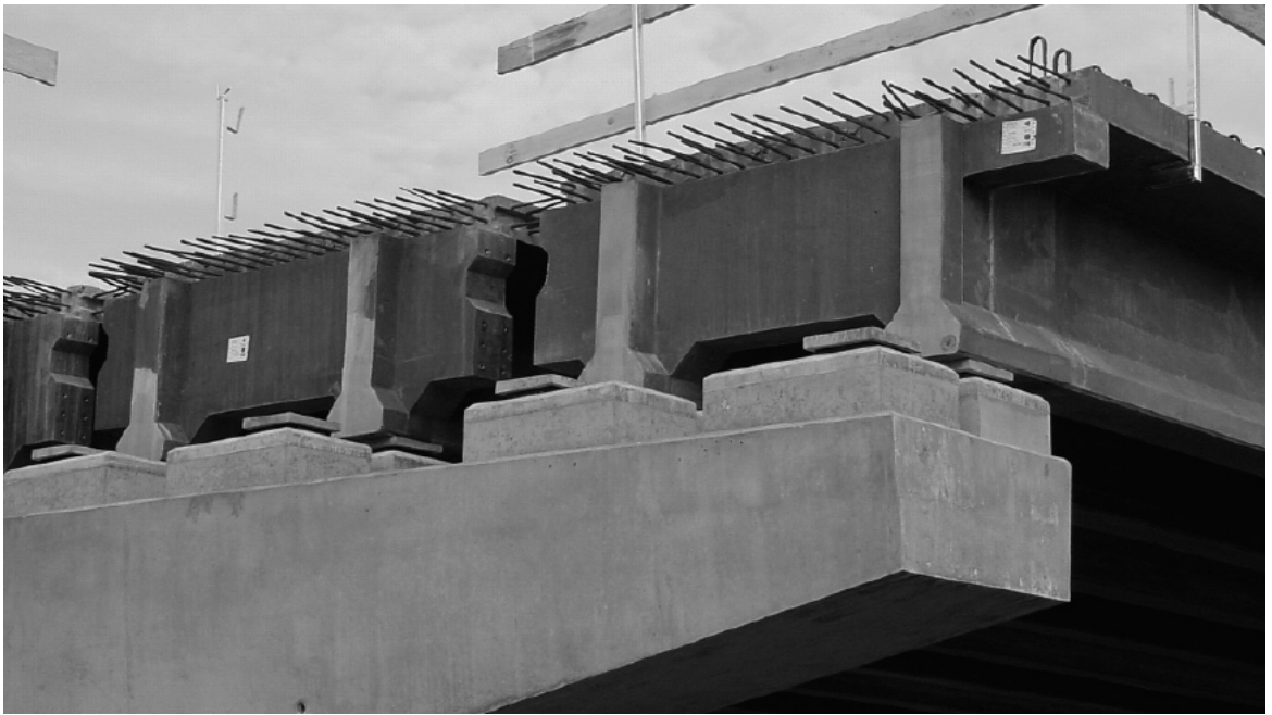
Figure 2.9: UHPC Pi-Girders in the Bourg-les-Valences Road Bridge in France (Vergoossen, 2008)
