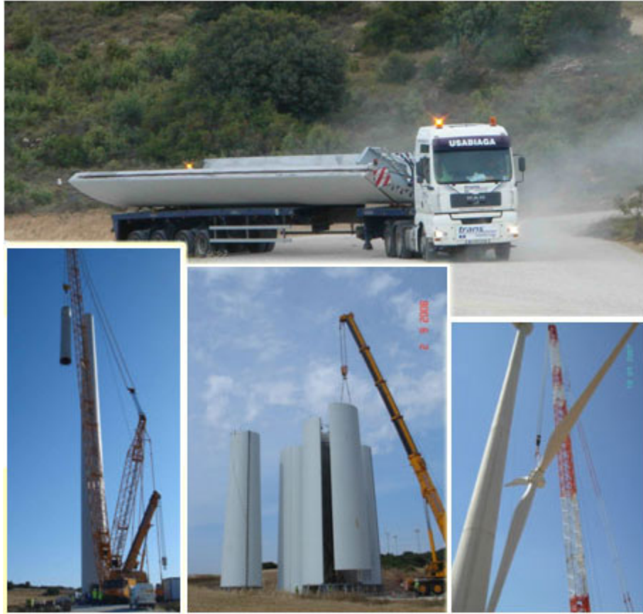
Figure 1.7: Precast Concrete Tower Transportation and Erection (Grupo Inneo, 2008)
