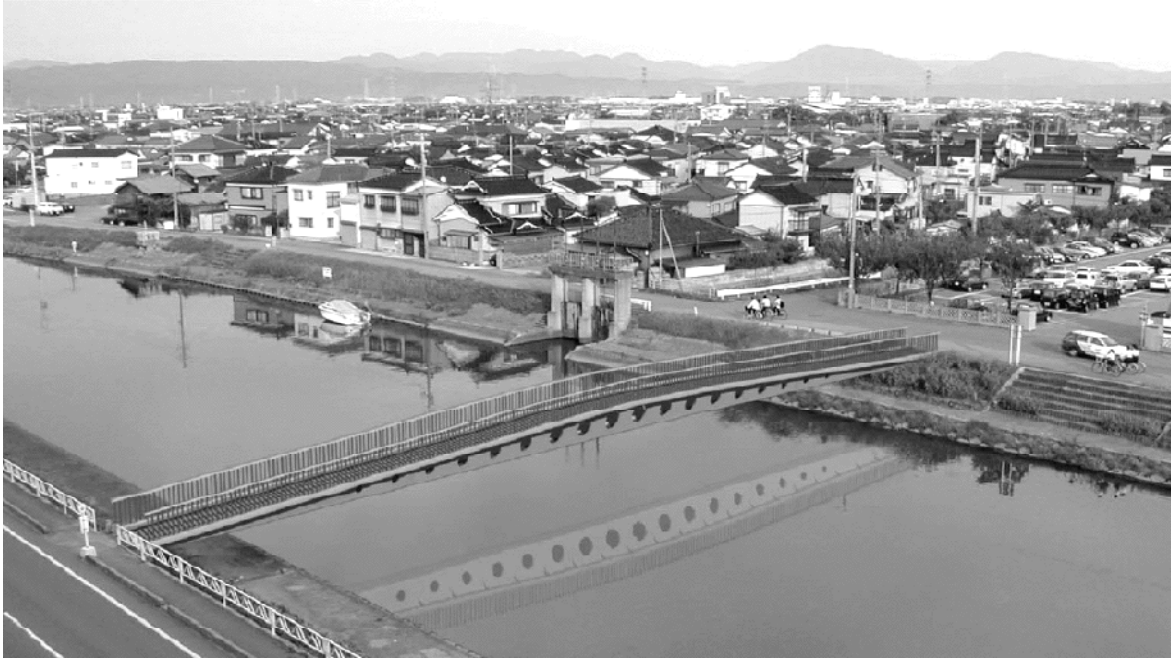
Figure 2.8: View of UHPC Sakata Mirai Footbridge in Japan (Tanaka et al., 2009)
