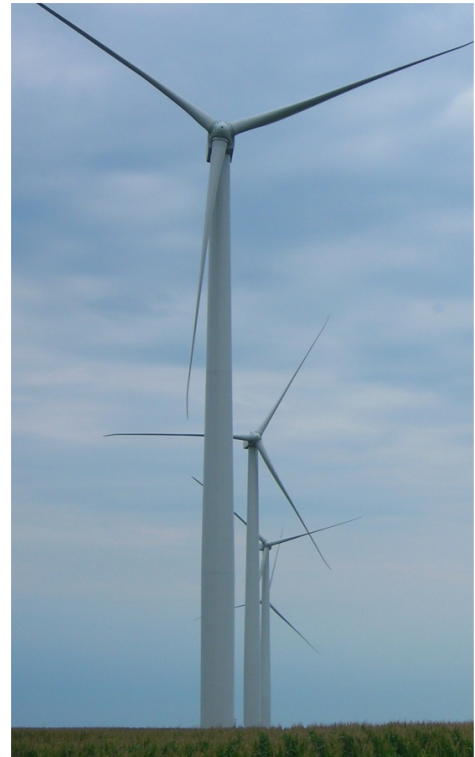
Figure 1.5: Steel Wind Turbine Tower
