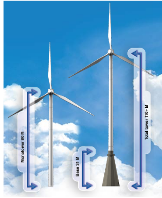
Figure 1.8: Illustration of the Tindall Atlas CTB Hybrid Tower (Tindall Corporation, 2009)
