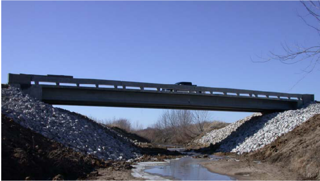
Figure 2.10: UHPC Mars Hill Bridge in Wapello County, Iowa (Keierleber et al., 2007)
